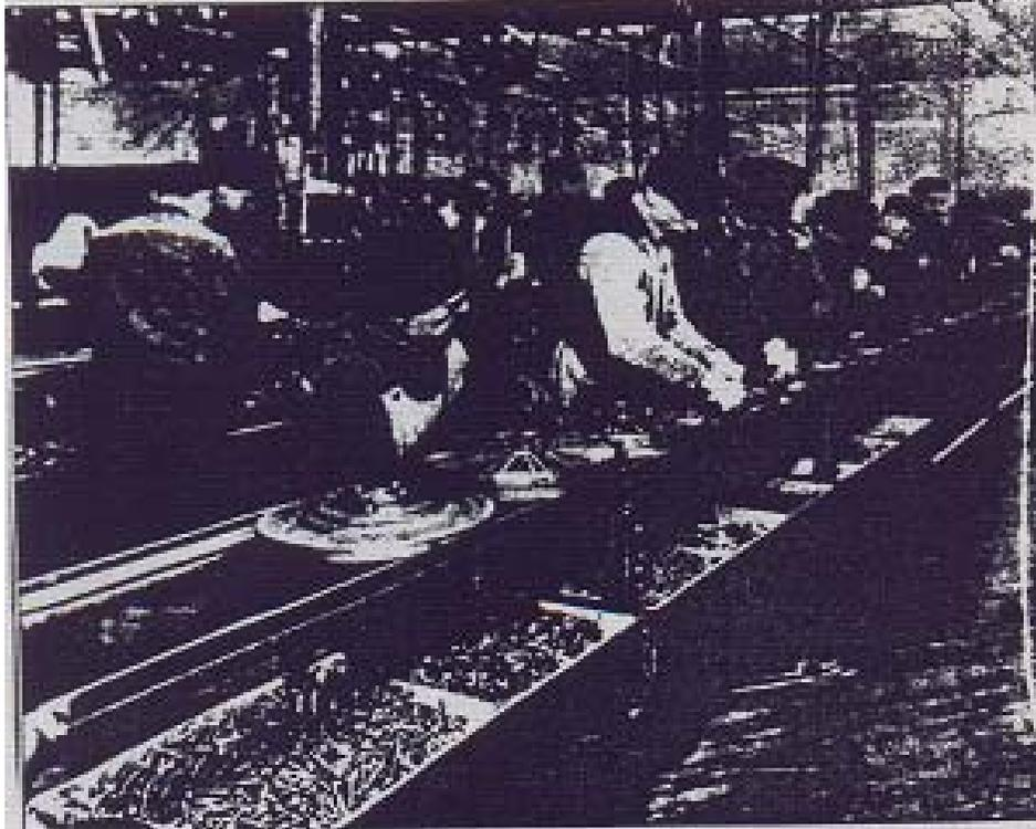
**Fig. 1. 2 Ford’s Highland Park Flywheel Magneto Assembly Line.**
